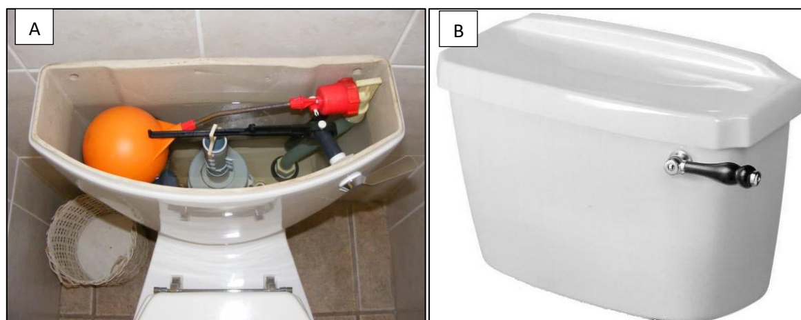
Figure 1: A: Standard flush mechanism, B: typical cistern
